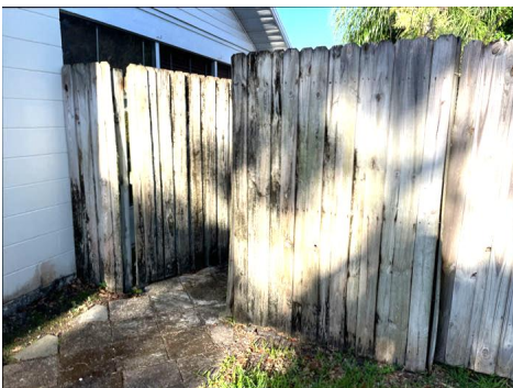
Fence were damaged.
