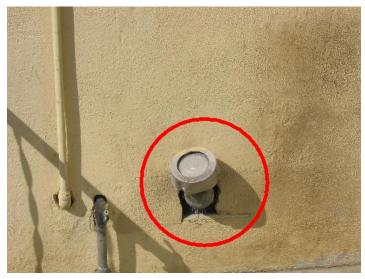
Improper installation of vent pipe. Exhaust vent from water heating in the basement area.
