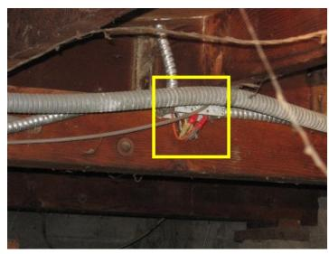
Exposed electrical connections. Missing junction box cover.
