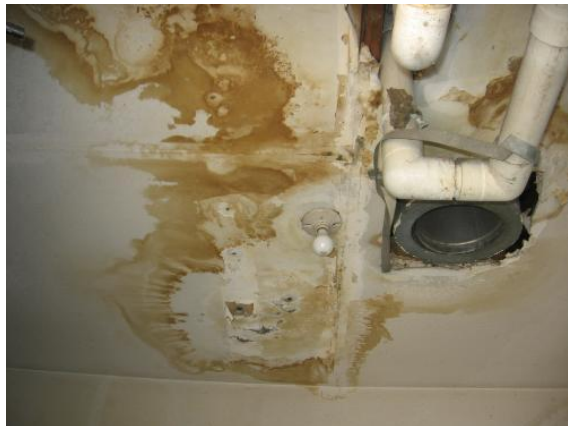
Pool - Equipment Room Ceiling
