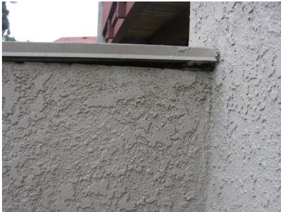
Grounds - Fencing and Walls
