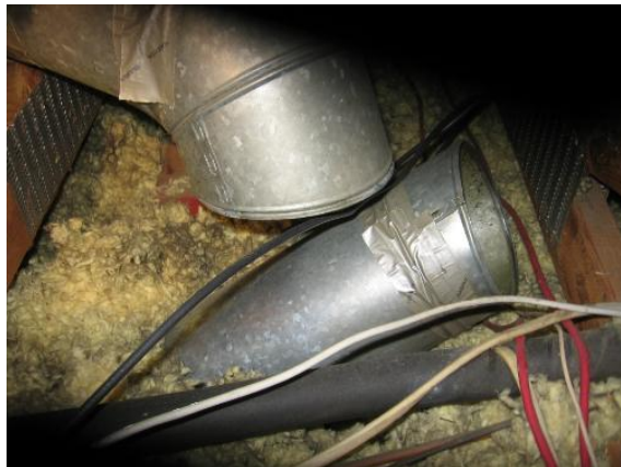
Attic - Exhaust Vent
