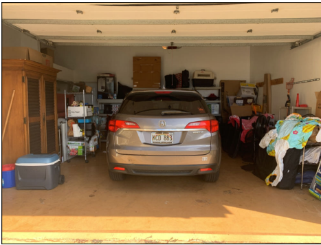
Attached 2 car garage.,Sectional door with motorized opener and safety sensors were tested and functioned normally.
