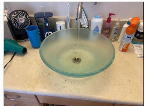
Slow drain accumulates water when in use. Repair. (Blue) Location: master bathroom.
