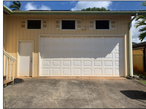
Front of garage.
