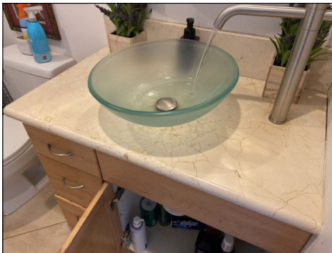
Sink fixture was unsecured to the countertop. Evaluate. Repair or replace as needed. (Red) Location: guest bathroom.
