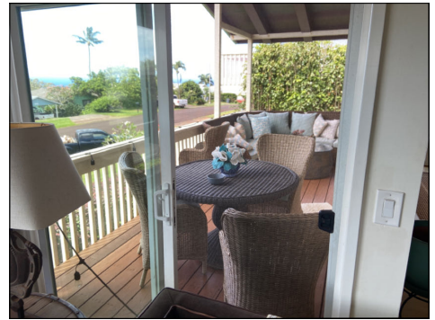
Sliding screen door(s) did not operate smoothly. Repair or replace as needed. (Blue) Location: living room.
