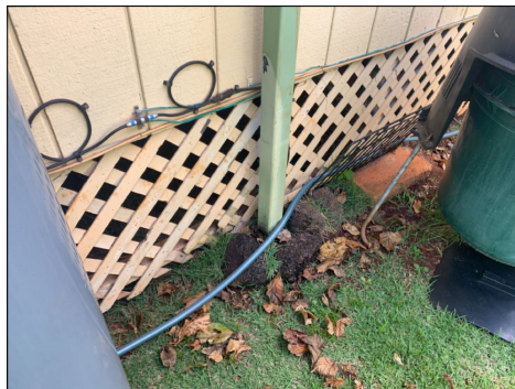
Remove debris from gutters to ensure proper function. (Red)
