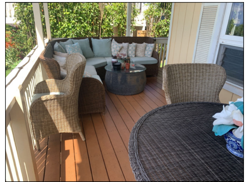
Deck/lanai description/location - Front of home. Surface/structure - Wood decking over wood joists. Handrails - Wood.
