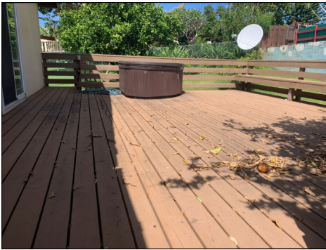
Deck/lanai description/location - Rear of home. Surface/structure - Wood decking over wood joists. Handrails - Wood.
