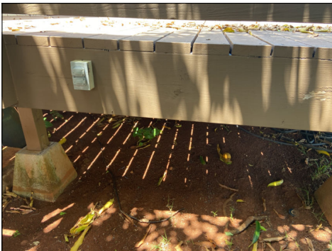
Foundation access. Location: rear of home below lanai.
