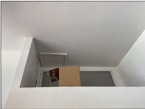
Attic access at Garage.
