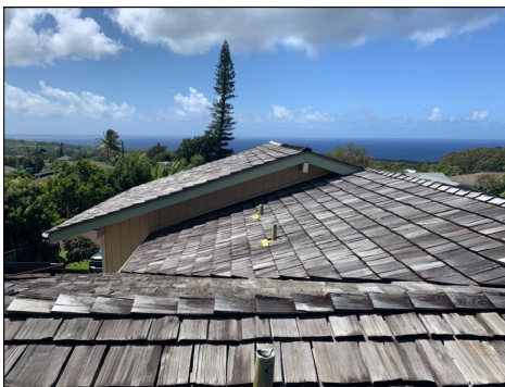
Roof inspection - Roof was walked. Roof materials - Wood shakes.
