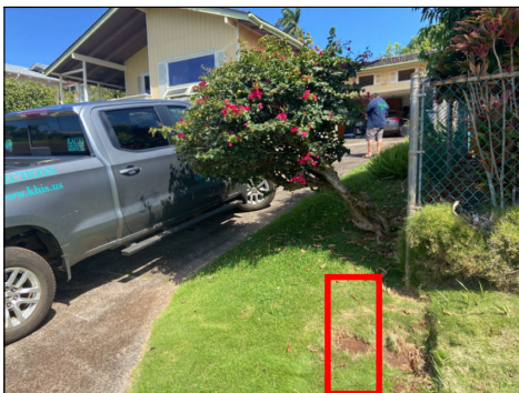
Water meter and main shutoff valve. Location: front of home.
