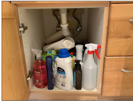
Personal belongings at master bathroom sink cabinet. Recommend review prior to closing to check for damages or defects.
